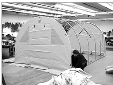
6) The spanners can now be installed. Again working from one end of the building toward the other, going one bay at a time, install the lower spanners first, then, top center.
