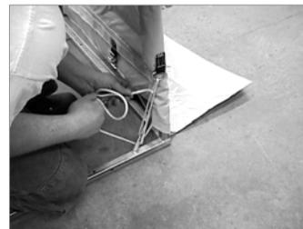
The panels have three cut-outs exposing the ¼" solid braid nylon rope that is sewn into a pocket hem. Start with the top center cut-out and slip the rope up and over the top center insert post. Move down to the lower insert posts and slip the rope over each. Snug up the rope so that the pocket hem gathers and raps toward the inside of the building over the frame. Move down to the bottom corners. Snug the rope.
